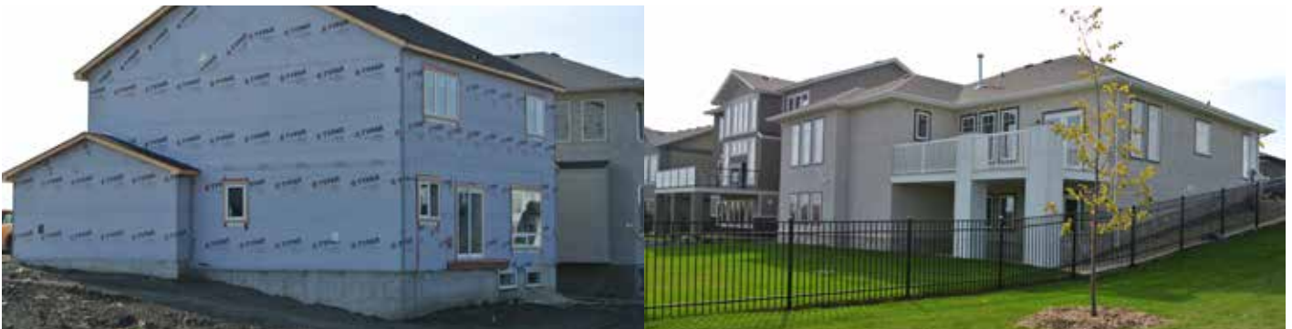
These photos show homes with a non-walkout design, and one with a walkout, providing access from the basement
