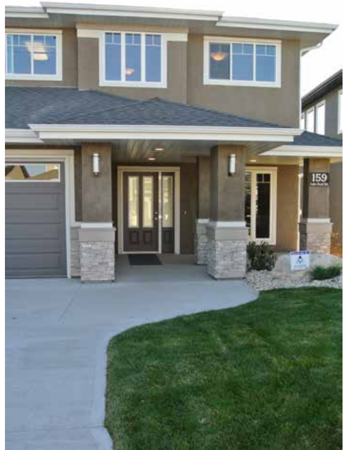
A front view of a Visitable home with a level threshold, level path to the side of the home and a wide entrance
