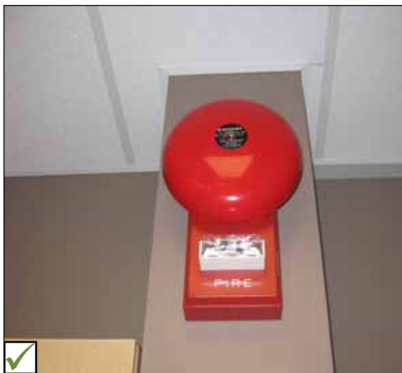
Example of combined visual and audible alarm signals. Public facilities should have both visual and audible fire alarm systems strategically located.
