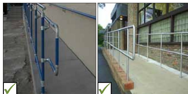
Figure 7b: Handrail Returns to Wall
